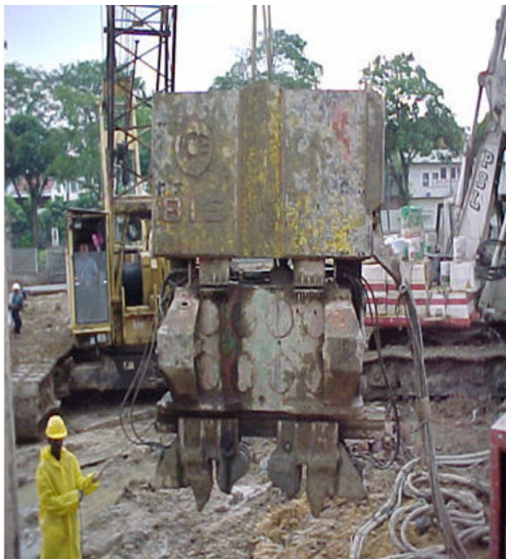
Figure 3-8 View of a vibro-hammer
