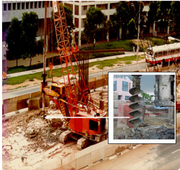
Figure 3-3 Pile installation by augering method
