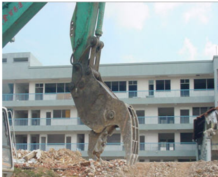
Figure 2-11 Use of a crusher for demolition helps to minimise the impact of vibration
