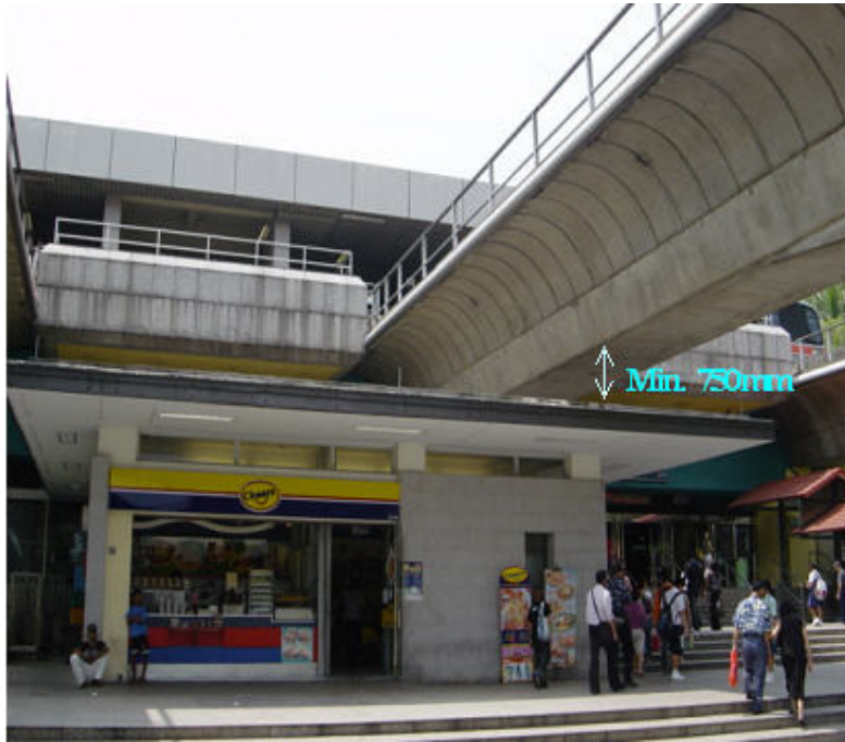
Figure 4-13 A convenience store located under the viaduct
