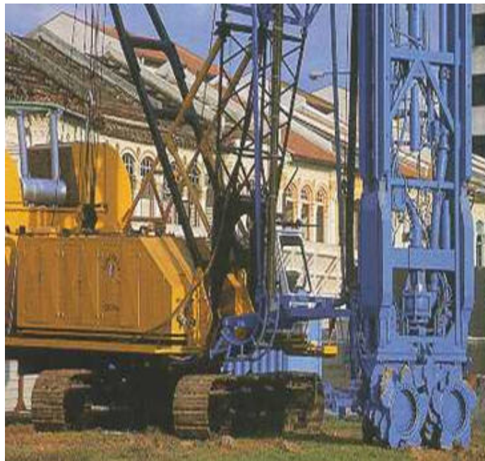
Figure 3-6 View of a hydrofraise machine
