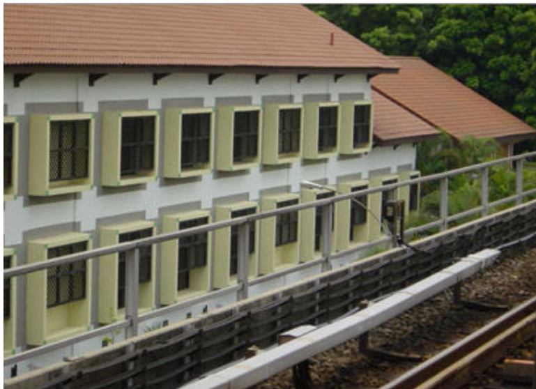
Figure 4-7 A multi-storey car park with facade opening facing the viaduct is provided with a protective screen
