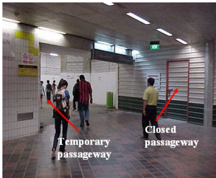
Figure 2-9 A safe and protected temporary passageway is provided during the construction of a commercial development
