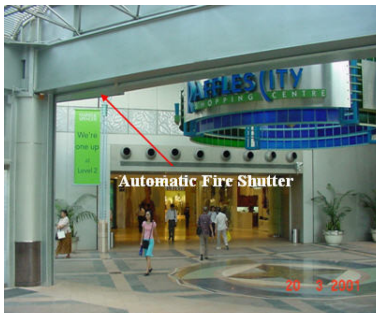
Figure 4-36 An automatic fire shutter at the interface between the commercial development and station entrance
