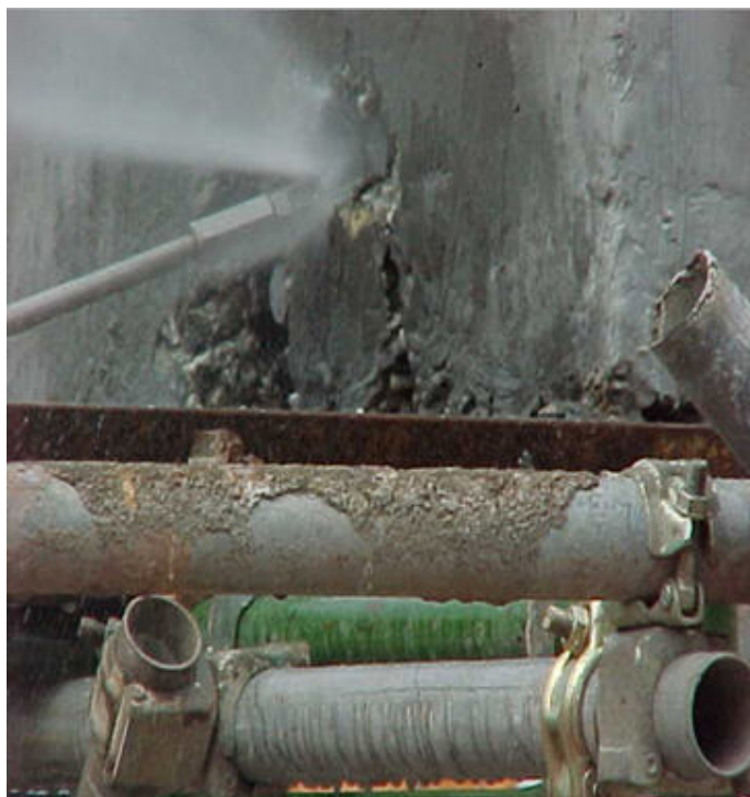
Figure 2-15 Use of a hydro-jet for demolition helps to minimise dust, fire hazard, vibration and noise levels
