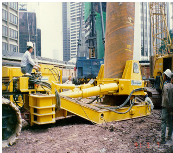
Figure 3-4 Pile installation by oscillatory method
