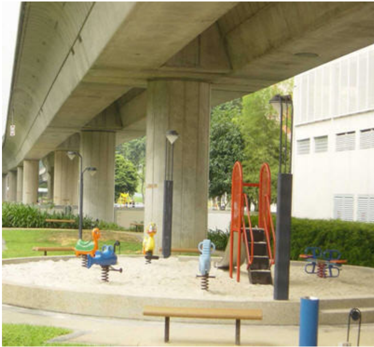
Figure 4-19 Land below the viaduct can be used to locate a children playground
