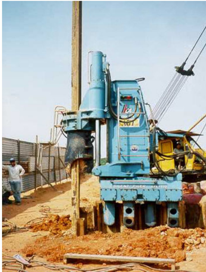
Figure 3-5 Sheetpile installation by a silent piler
