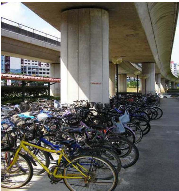
Figure 4-20 Land below the viaduct can be used to locate a bicycle park
