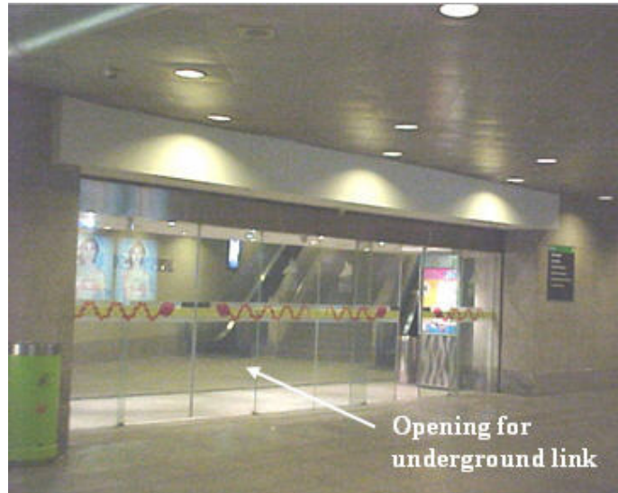
Figure 6-3 An opening created in the wall at concourse level of Bugis Station
