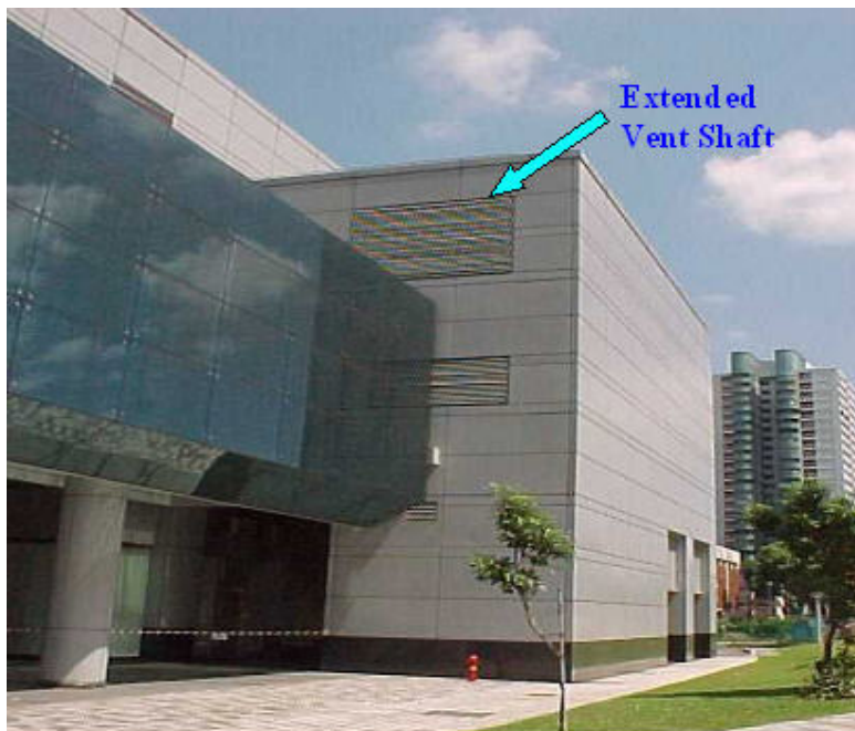
Figure 4-29 Building with RTS ventilation shaft extended from the existing one at ground level
