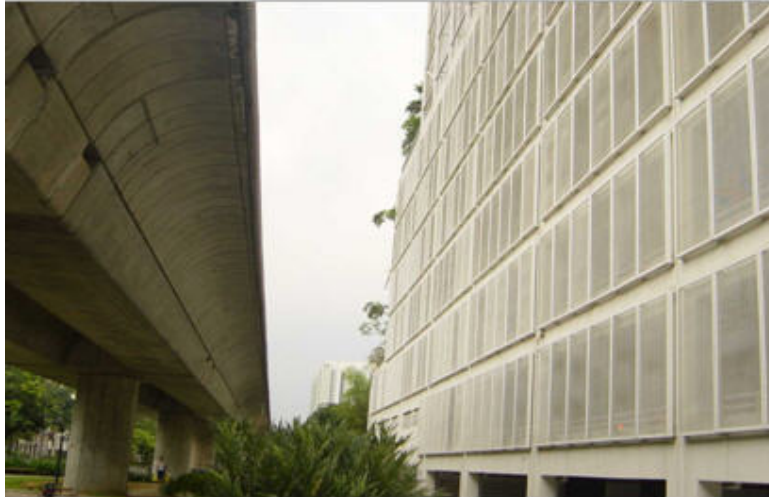
Figure 4-6 A multi-storey car park with facade opening facing the viaduct is provided with a protective screen
