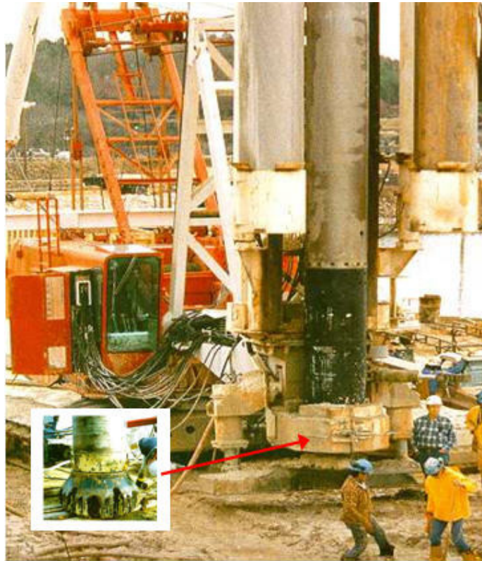
Figure 3-7 Pile installation by down-the-hole drilling technique
